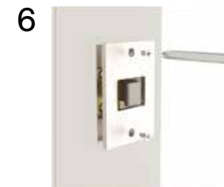
6 Mount cuff Mount the bolt cuff aligning per template Install trim accordingly
