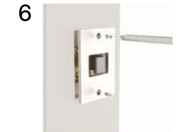
6 Mount cuff Mount the bolt cuff aligning per template Install trim accordingly
