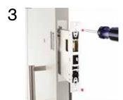
Insert lock into door Insert lock into door
